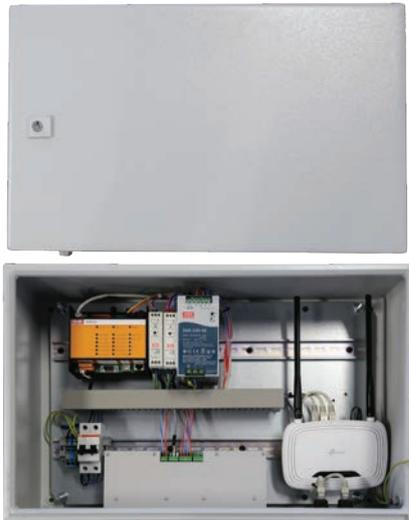
The central control cabinet of the EVC system is used for connection of room / zone HUBs, as well as an interface to the air handling unit control and the building control system.
