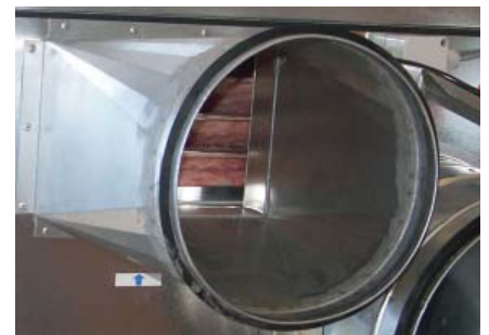
Adapter set OKM, suspension device and vibration dampers
